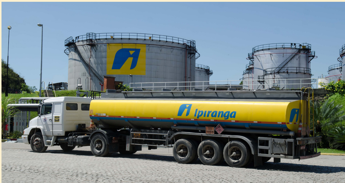
Figure 1: Ipiranga Fuel Distribution Base
